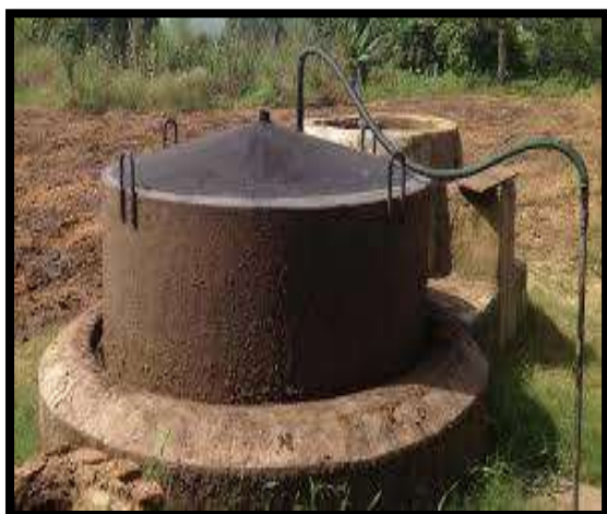
Fig. 3.9 BIO GAS PLANT
